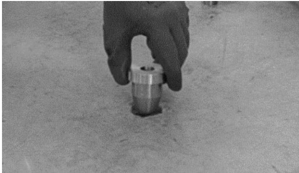
Figure 3. Testing Depth with the Drilling Guide
